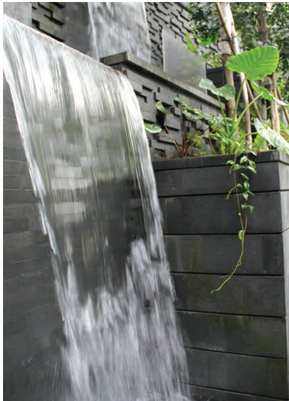
The walls of the waterfall are covered with lava stone slabs installed with KERAFLEX MAXI S1. The joints were grouted with KERACOLOR SF.
