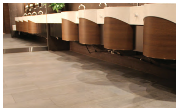
The granite in the bathrooms was bonded with GRANIRAPID and grouted with KERACOLOR SF. The substrates were treated with PRIMER G before bonding the granite.
